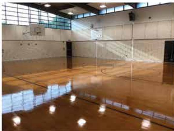
Refinished Gym Floor
