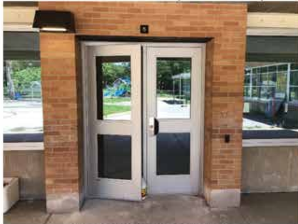
Exterior Door Installation
