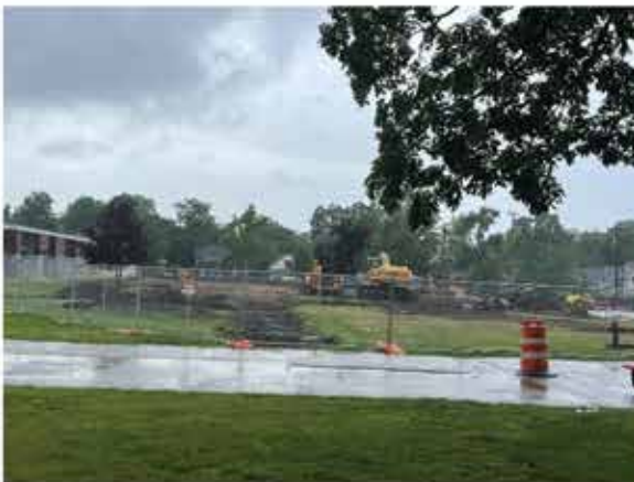
Parking Lot Work
