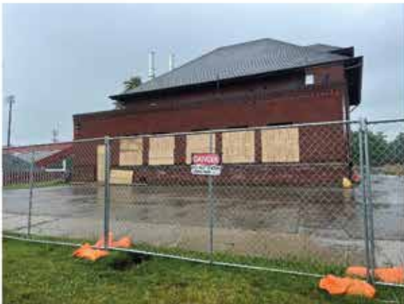
Prepped to Begin Demo
