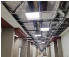
1st Floor Classroom Wing Ceiling
