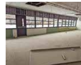
Interior Framing & Wall Prep
