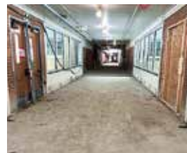
Hallway Floor Demo
