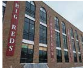
South Elevation Exterior
