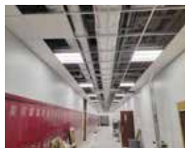
Corridor Lights and Ceilings
