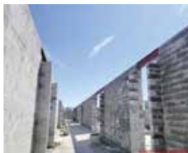
3rd Floor Classroom Bearing Walls
