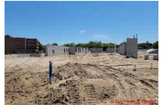
Backfilled Plumbing
