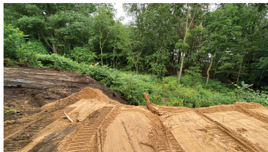
Norse Nature Preserve ADA ramp prepping.
